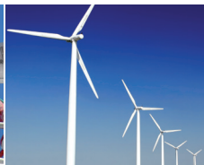
Wind Park Monitoring / SCADA
